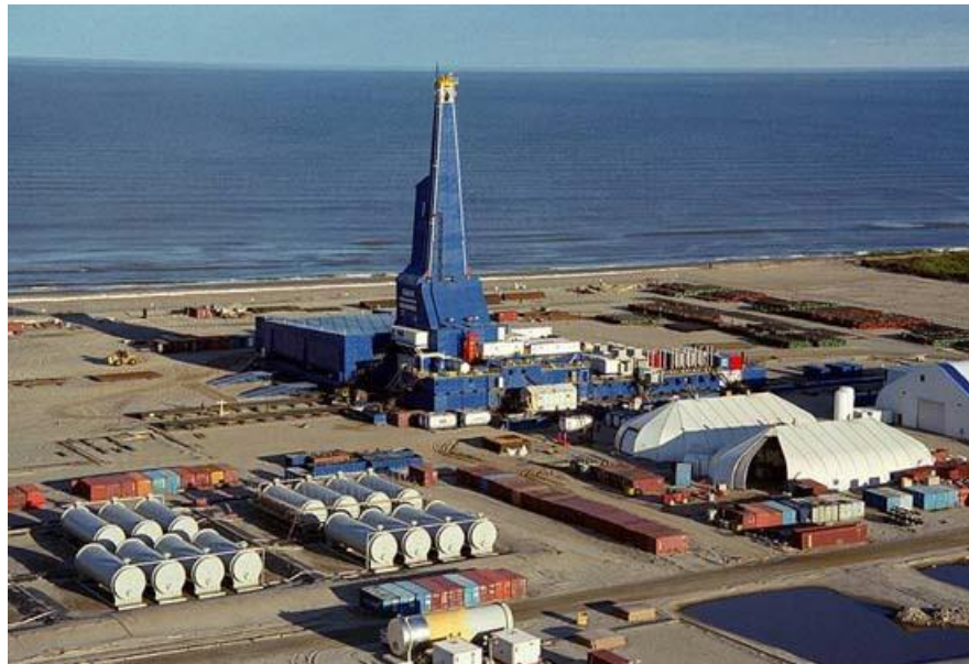
The Chayvo Yastreb land rig is the research center and testing site for the Z-44 Chayvo Oil Well, the deepest hole ever drilled into the earth.
