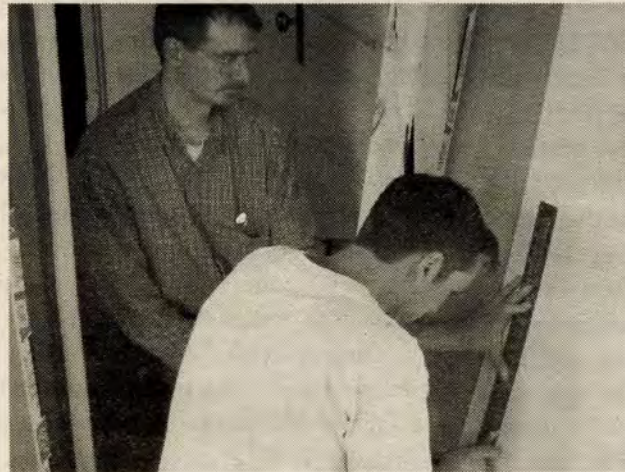
KRFP volunteers hard at work renovating the new station.
