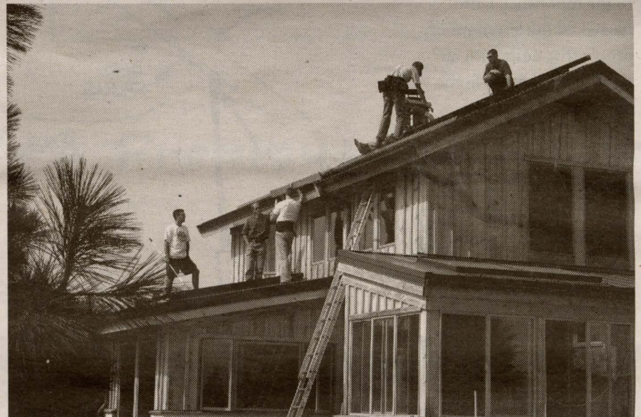
The Forbes family home in progress.
