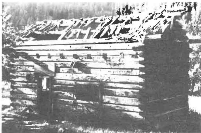
Jim Moore house (before stabilization).
